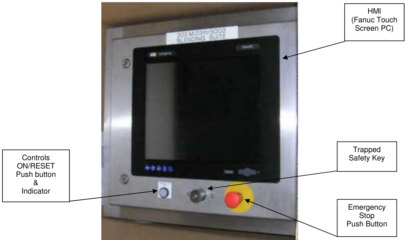
Fig 17 - IBC Blender Suite – Operator Control Panel
