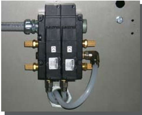
figure 58-1. Parker Hanafin Valve Bank
