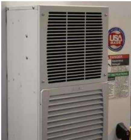
Industrial Air Conditioner "Electrical Cabinet"
