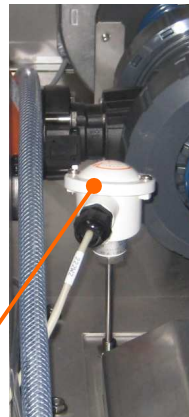
PT100 sensor with built-in converter ( at the top )
