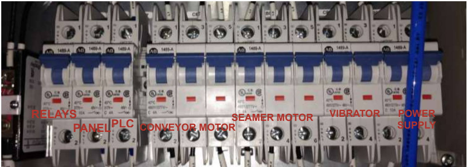
Figure 11 Top row of breakers
