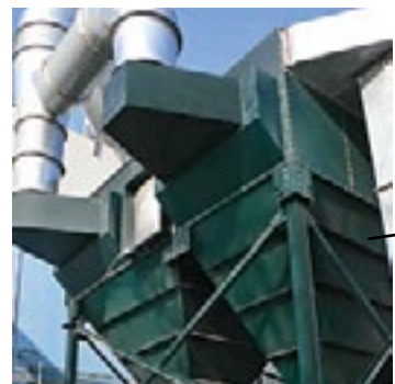
High Entry Inlet Cross flow is created through the filters. This eliminates upward “can” velocities associated with traditional hopper inlets.
