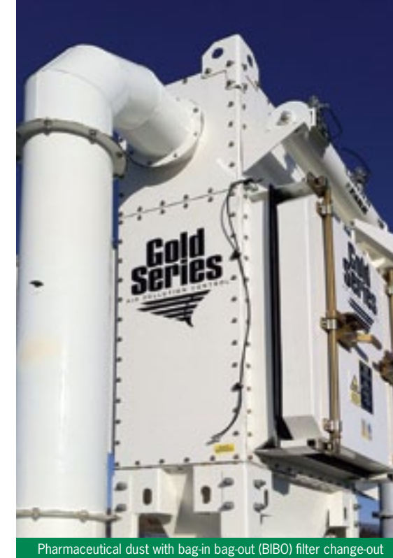
Pharmaceutical dust with bag-in bag-out (BIBO) filter change-out
