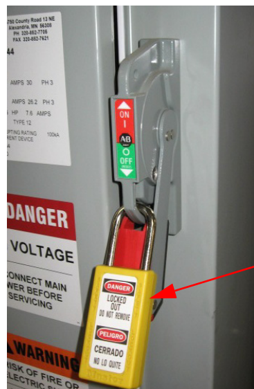
Figure 1 - 3 Electrical Lock Out
